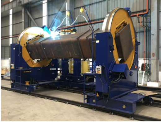
Robot Column Welding 15 Ton
